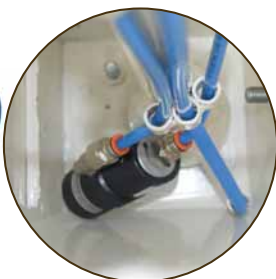
WINDOW TO CONTROL AND UNLOAD THE RESIDUAL POWDER AND VIBRATING SYSTEM
